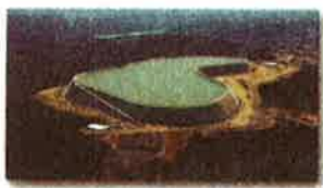
The Taum Sauk Upper Reservoir Dam is located on the east fork of the Black River in Missouri. The project was named the ESWP 2010 Civil Project of the Year.
